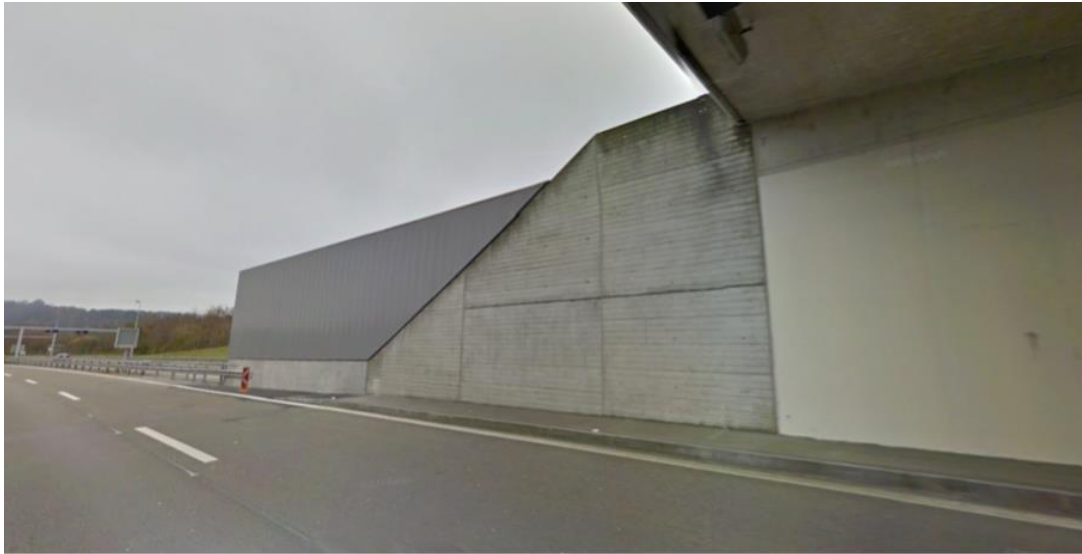
Figure 12: Dividing Wall at Tunnel Portal
