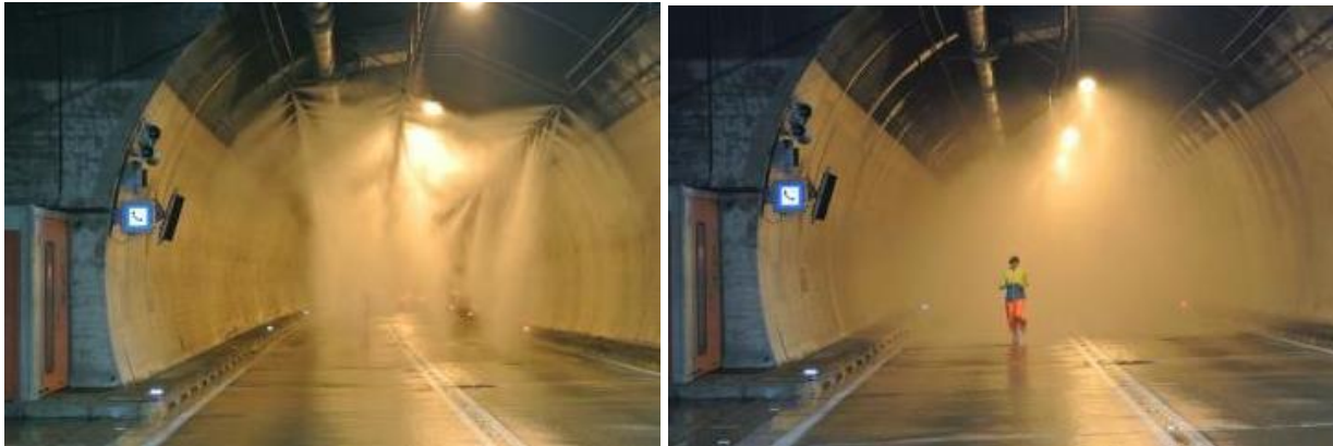
Figure 11: Test Activation of Water Mist FFFS in a Road Tunnel
